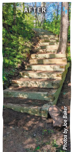
Contractor North Country Trailbuilding led volunteers in projects around Skyline including building these cribbed steps.
