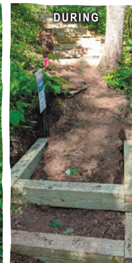
Contractor North Country Trailbuilding led volunteers in projects around Skyline including building these cribbed steps.
