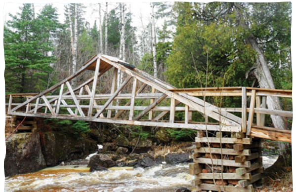
Old Split Rock River Bridge.
