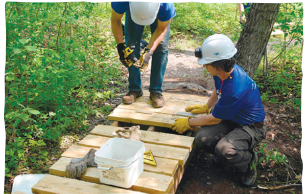
Volunteers from Minnesota Power building puncheon in Duluth during the 2025 United Way Day of Caring.
