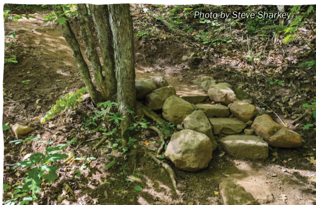
On the main trail portion of the Bean and Bear Lakes Loop contractors used locally sourced materials (rock) to design resilient and dramatic stone steps.
