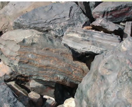
Bedded taconite riprap, Lakewalk
