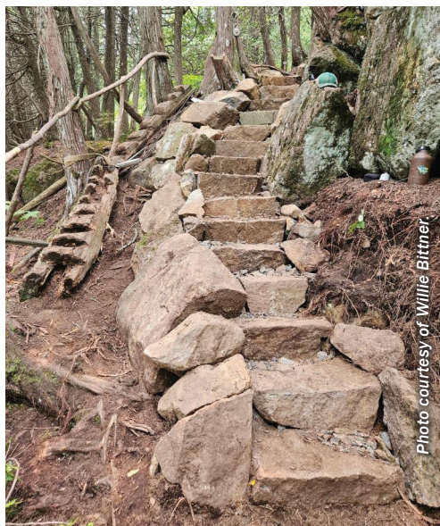
On the left, the old notched log stairway rests next to a wonder of stonework by contractor Willie Bittner of Great Lakes Trailbuilders, LLC with a field crew from the Conservation Corps of Minnesota & Iowa.
