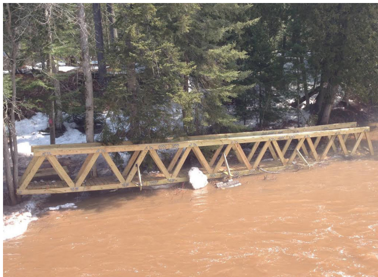
The bridge washed out during 2013's spring melt. It was time to move to a different crossing method — stone steps!
