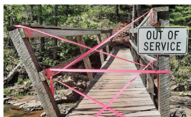
The Indian Camp Creek bridge was permanently closed by the U.S. Forest Service after damage from the 2022 spring melt floods made it unsafe. Photo courtesy of Cathy Quinn, USFS.
