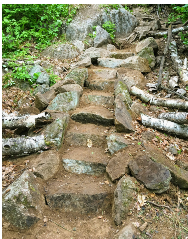
Stone staircases like this one near Bean and Bear Lake will be increasingly used when rock is available on site.
