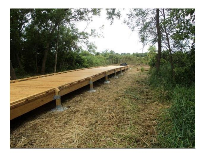
This second example shows a similar structure, built with the same footings, in a flooded area. It was, however, built in dry conditions when no water was present. Another possibility, which may be better suited to this application would be the use of helical piers. Information on galvanized steel footings (Bog Pans) can be found at: <a href="https://custommfginc.com/">https://custommfginc.com/</a>
