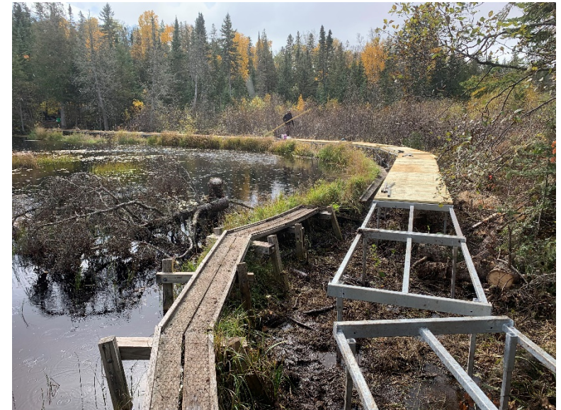
Before & after of old Boardwalk being replaced with longer lasting and safer material.
